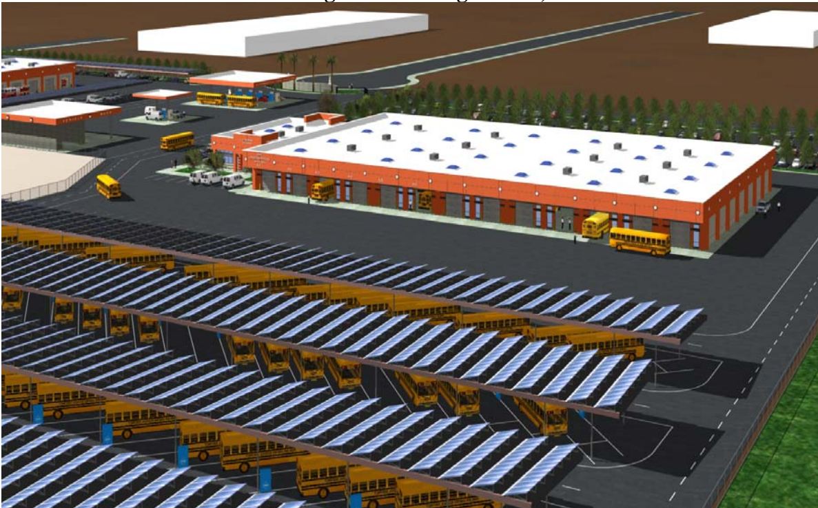
Figure 2: Fueling Station, Aerial View
