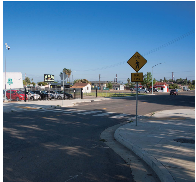
Mid-block crosswalk with bulb outs in Orange Cove
