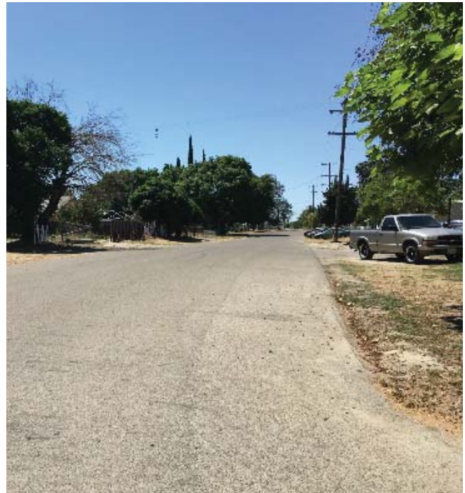
Street lacking sidewalks, curbs and gutters in the unincorporated community of Raisin City
