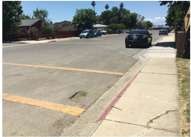
Crosswalk near Huron Elementary School that lacks adequate curb ramps
