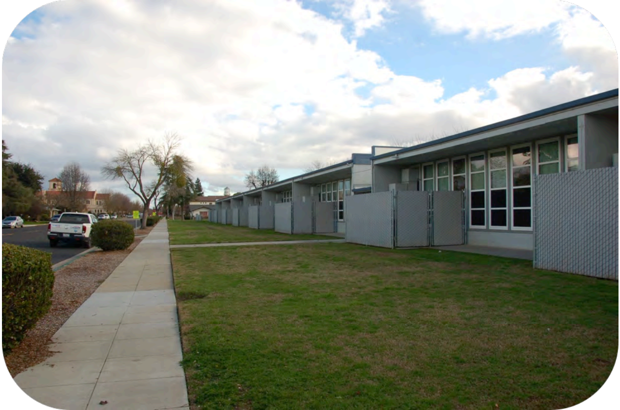
Fremont Elementary School
