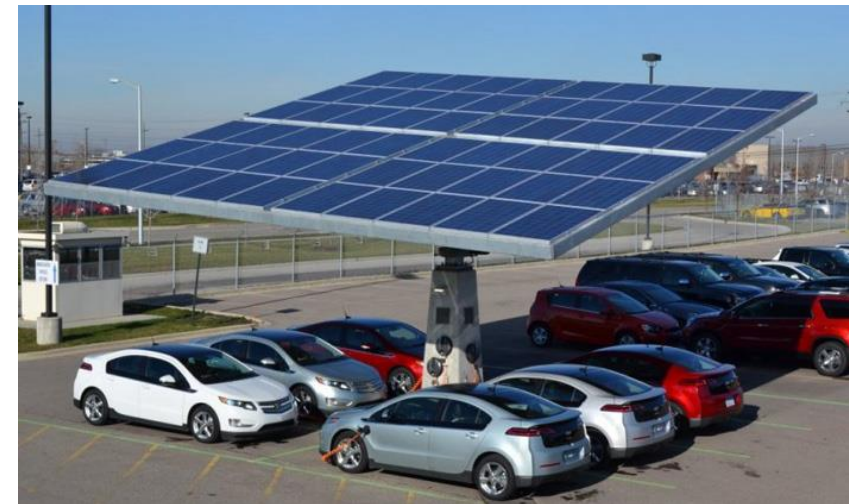
EV Solar Tree Charging Unit
