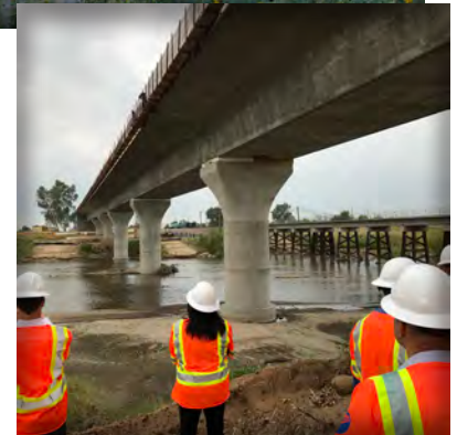
Above: The Cedar Avenue Viaduct will carry high-speed trains over Highway 99 before descending into the station area in Downtown Fresno.
