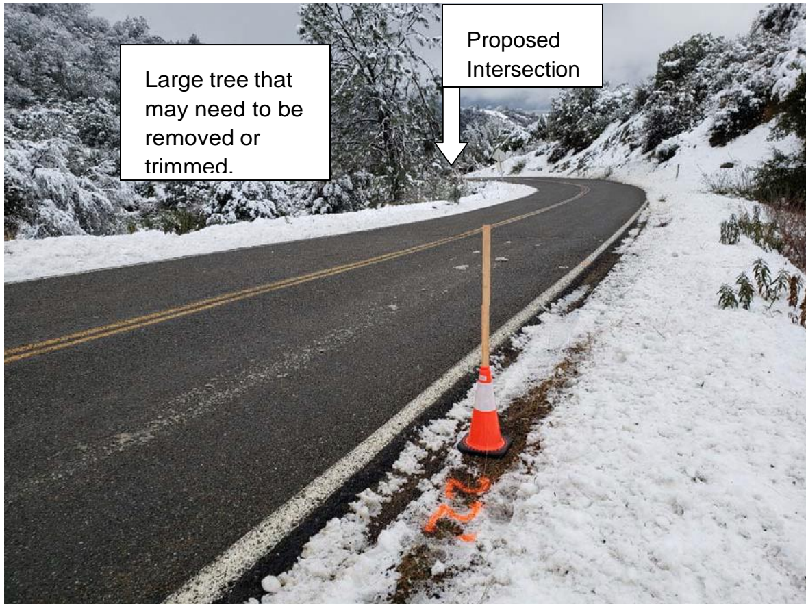
Figure 2- Sight distance measurement to the left of the intersection.
