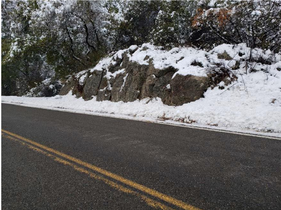
Figure 5 - Rock outcropping to be trimmed to improve sight distance.
