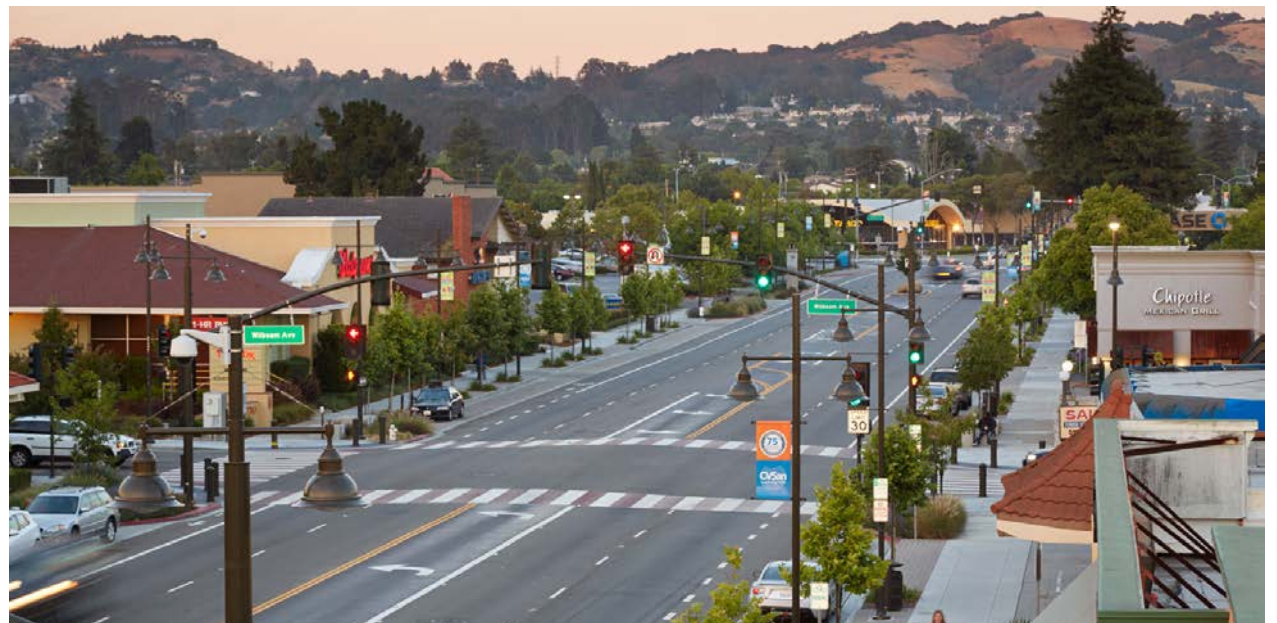
Right of way improvements with reduced traffic lanes, added bike lanes, clearly marked pedestrian crosswalks and wide sidewalk with retail frontages.
