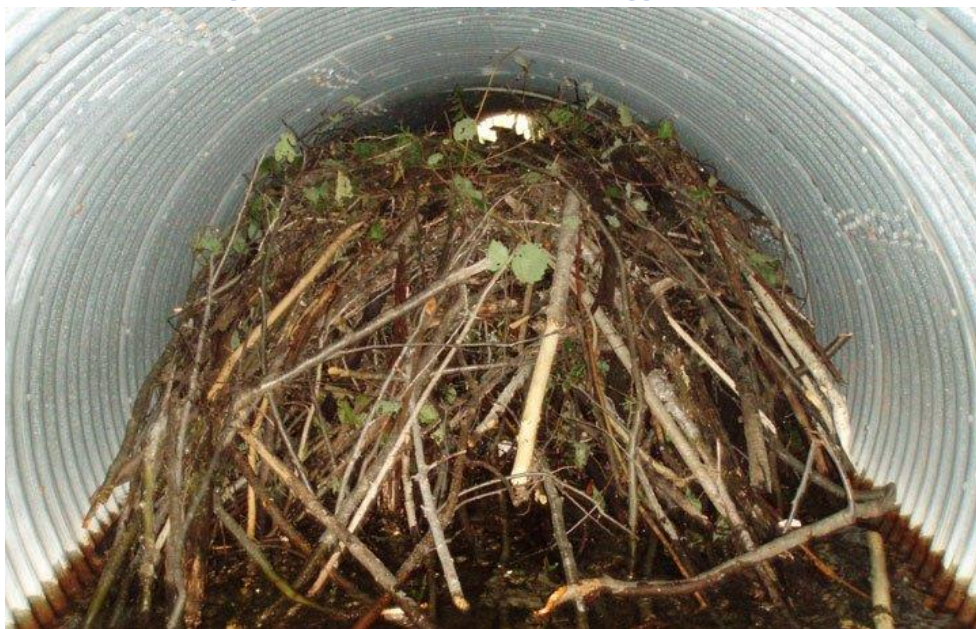
Figure 12: Caltrans District 10 Clogged Culvert
