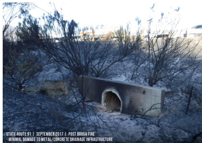
Figure 21: Metal Pipe and Concrete Headwall Post-Fire
