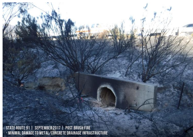
Figure 21: Metal Pipe and Concrete Headwall Post-Fire
