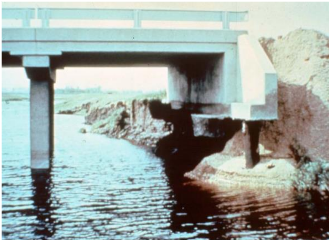
Figure 13: Bridge Abutment Scour
