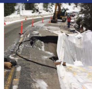
Washout on SR-41, photo courtesy of Caltrans
