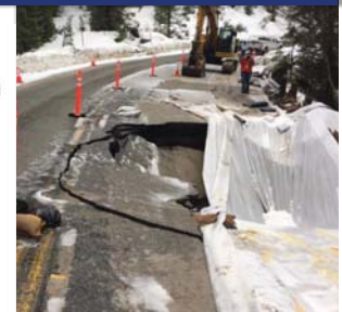
Washout on SR-41, photo courtesy of Caltrans
