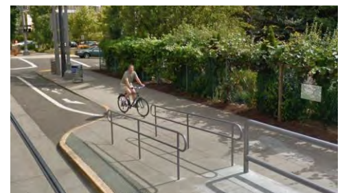
Figure 25: A separated bike lane transitioning to from on street to shared path/sidewalk behind a transit stop.
