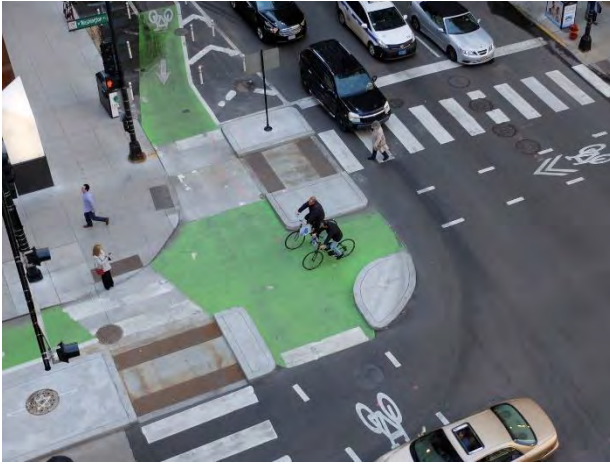
Figure 20: A separated bike lane in an intersection (left), and a graphic of a bicycle signal to protect bicyclists from right-turning traffic (right).
