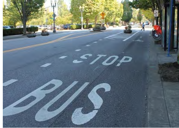
Figure 22: Unprotected mixing zone between separated bike lane and transit stop.
