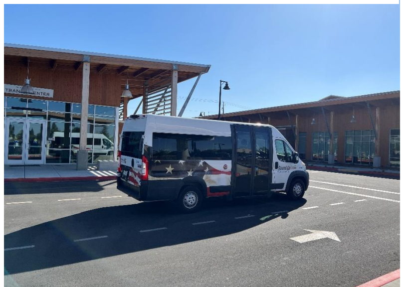
Figure 20 The Landmark Transit Center in Clovis is a recently constructed hub for bus and paratransit service and could be an ideal mobility hub site with proximity to Old Town.
