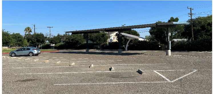
The Parlier Police Station west-side parking lot, where the mobility hub would be located.
