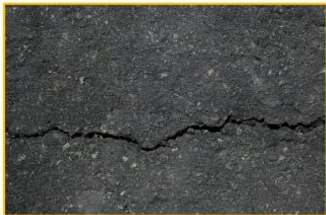
Heat-vulnerable pavement of roads
