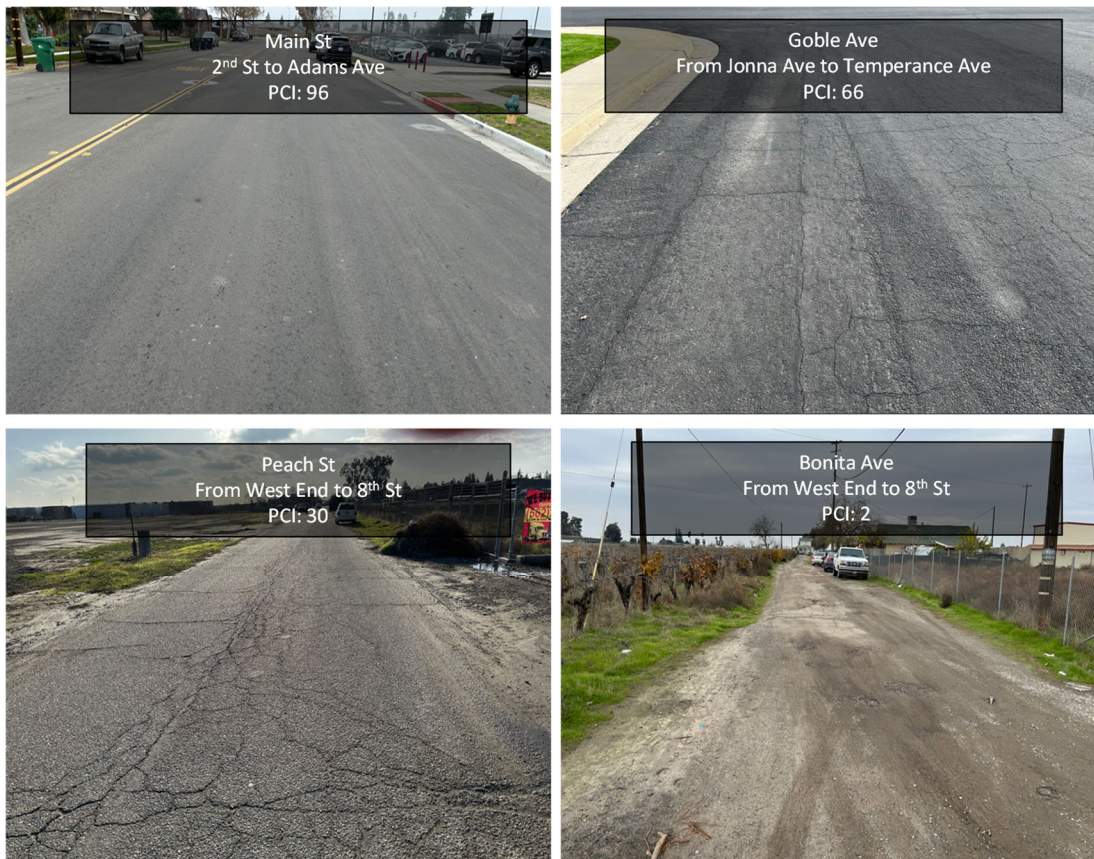
Figure 1. Examples of Streets with Different PCIs.
