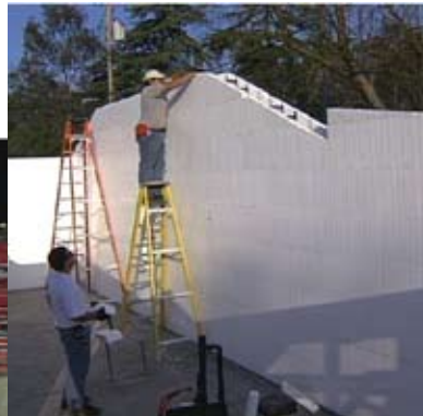
Tubing for Radiant Flooring (left); Installation of Insulated Concrete Forms (right)
