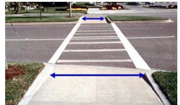
The images above show a high-visibility crossing at an intersection. The median has a curb cut through it to facilitate crossings. On streets with no medians, short islands like the one below provide refuge for people crossing where there are no signals.
