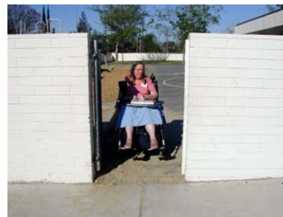
A wheelchair cannot negotiate this entrance to the school grounds because there is a depressed dirt area separating the asphalt on one side of the wall and the concrete on the other side. Neither children nor someone in a wheelchair can see over this wall to determine if it is safe to enter. The area near the school lacks curb ramps and continuous sidewalks.
