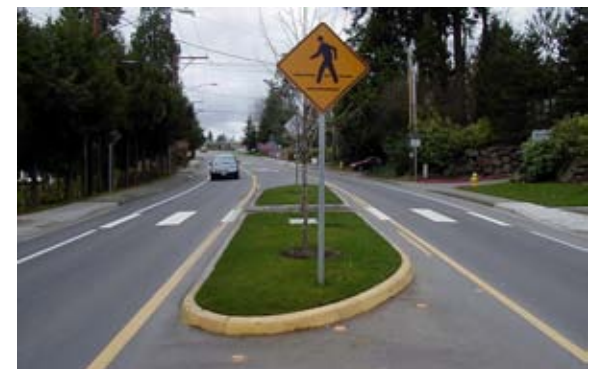
The images above show a high-visibility crossing at an intersection. The median has a curb cut through it to facilitate crossings. On streets with no medians, short islands like the one below provide refuge for people crossing where there are no signals.
