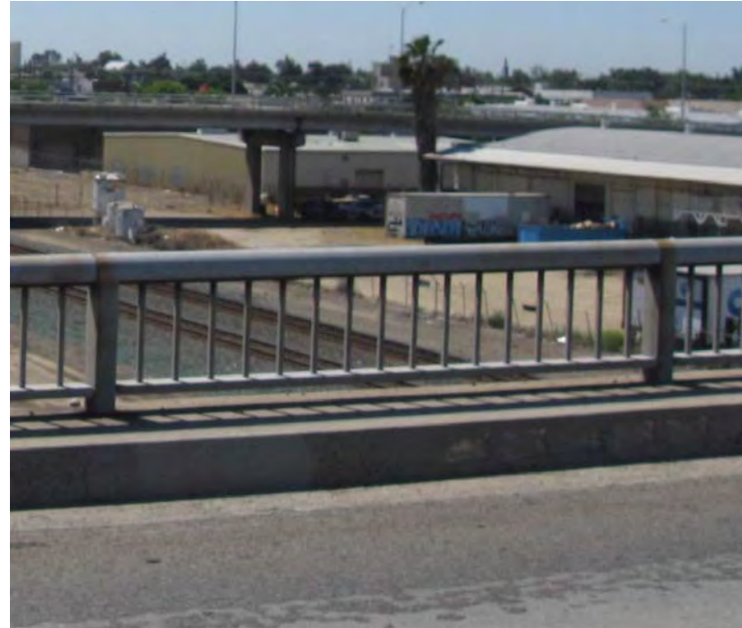
Example: Existing railing on Stanislaus Bridge that does not meet current code
