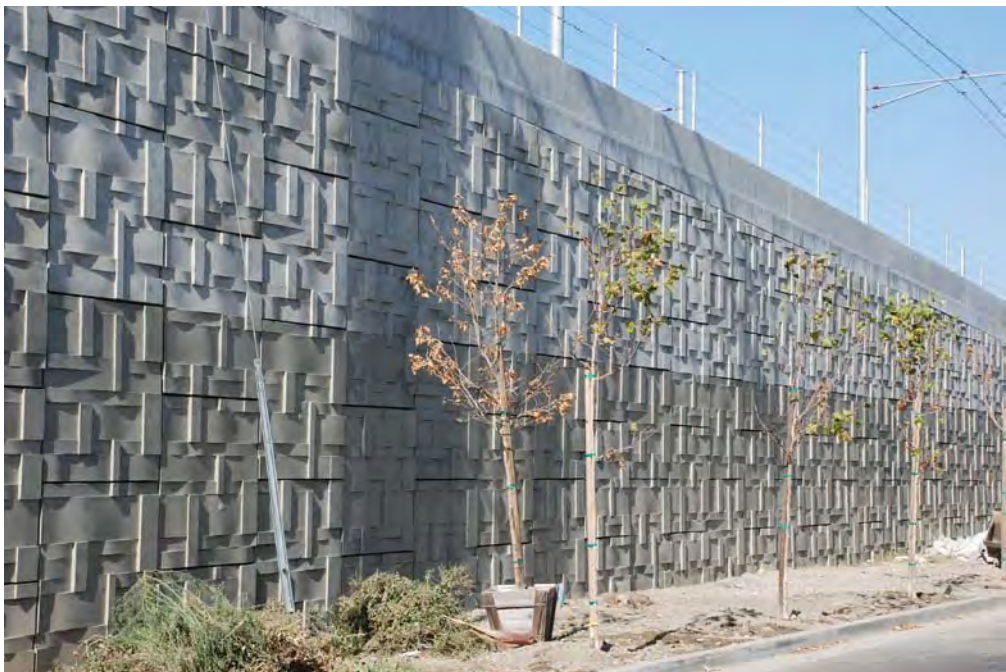
Example: MSE Fill Wall with custom texture
