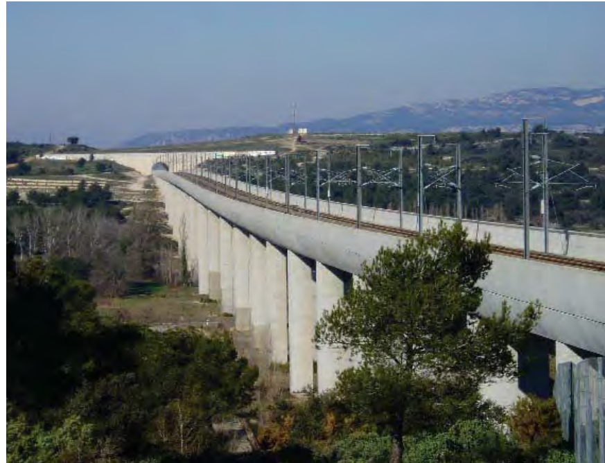
Example: Integrated concrete parapet HSR guideway
