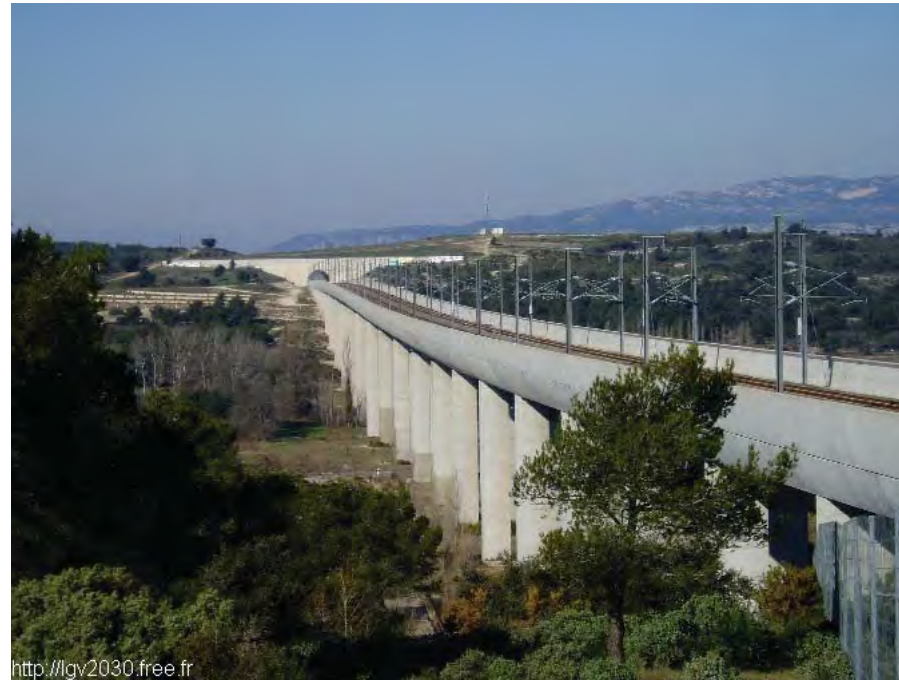
Example: Integrated viaduct and rounded parapet barrier
