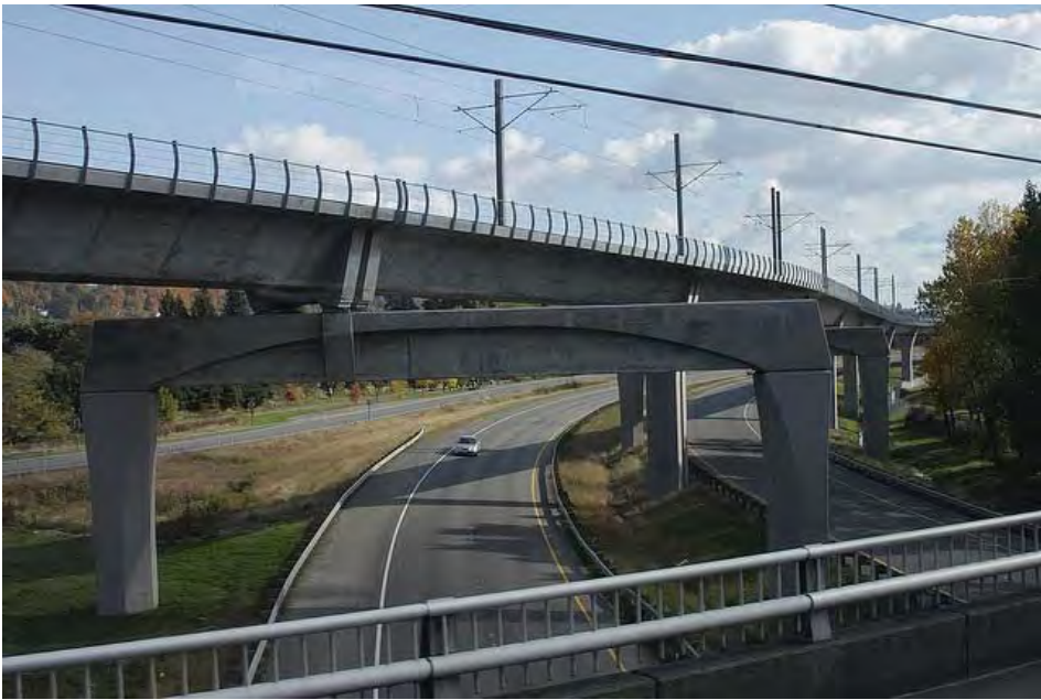
Example: Straddle bents over two roadways
