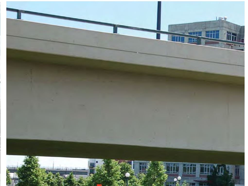
Example: Combination concrete parapet with metal tube railing
