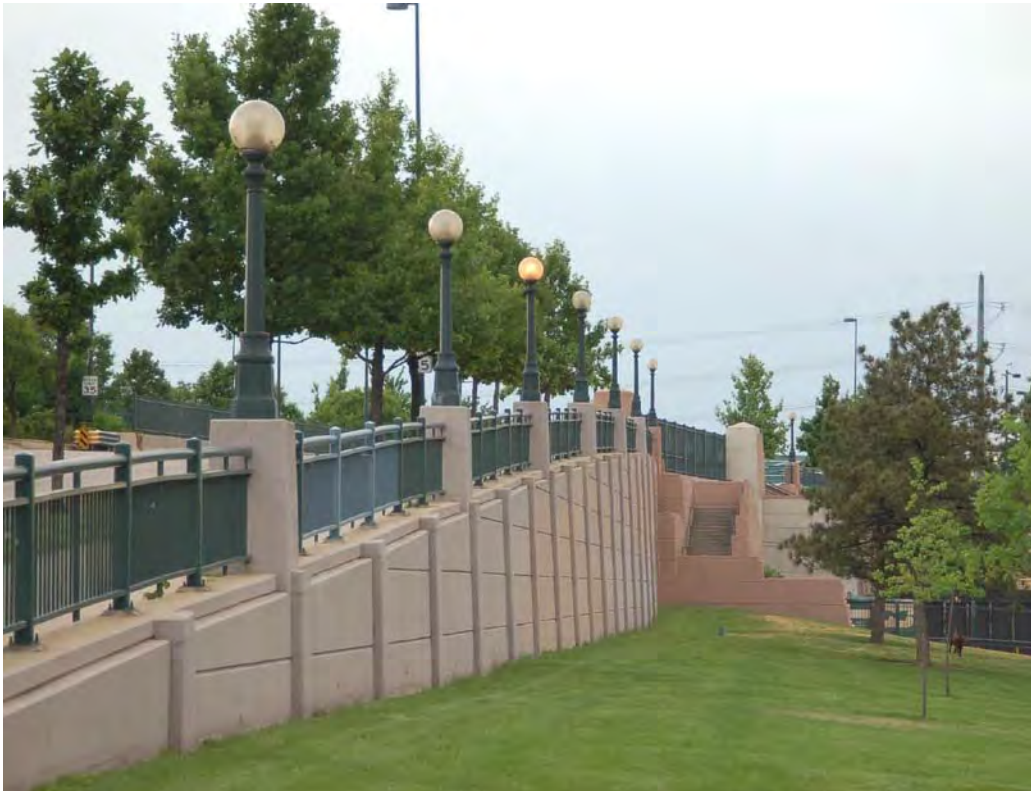
Example: Cast-in-place wall with architectural modulation
