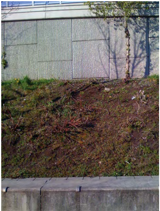
Example: MSE wall with fractured fin finish
