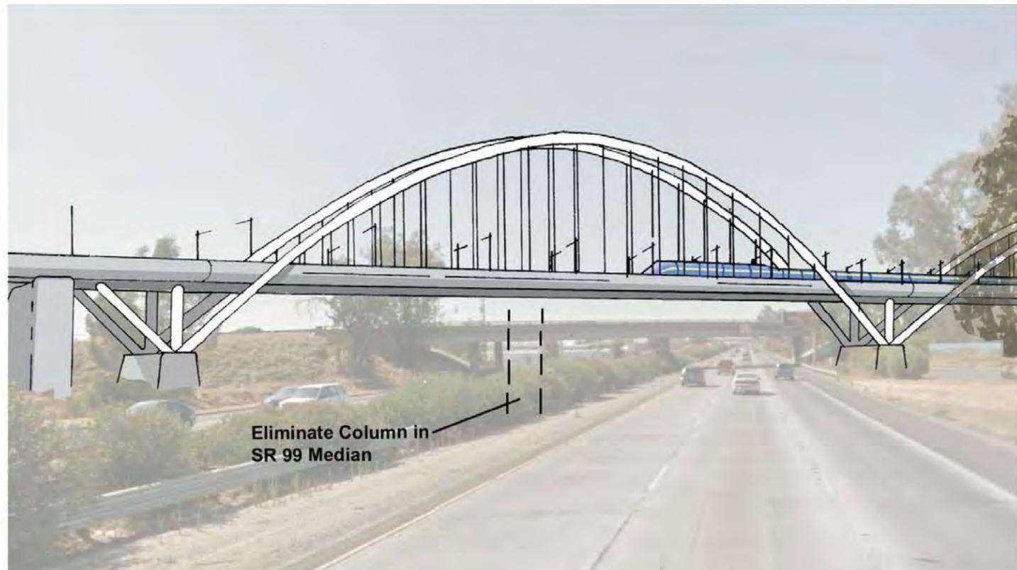
Recommendation: A single through-arch over Highway 99, with a smaller through-arch over Cedar Avenue.
