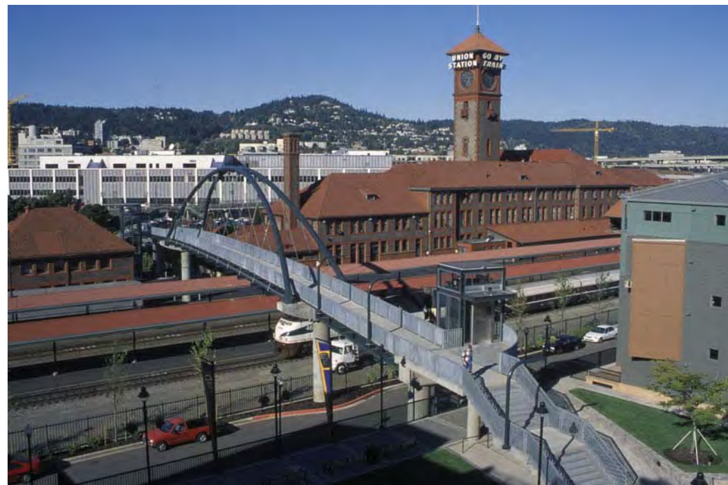
Example: pedestrian bridge over active rail tracks
