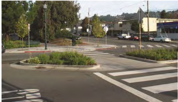
Pedestrian refuge island and striped crosswalk
