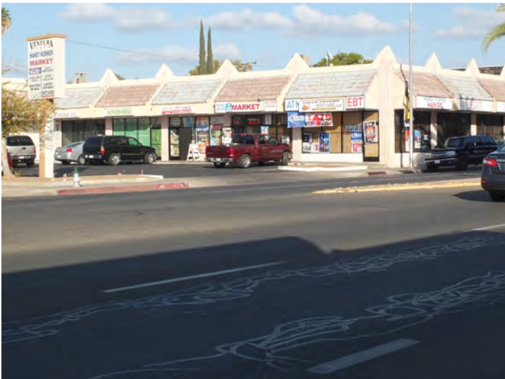
Crosswalk Location (before)
