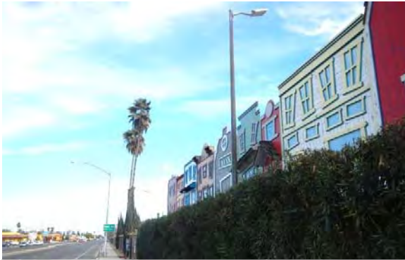
Decorative facades at street edge of Fairgrounds
