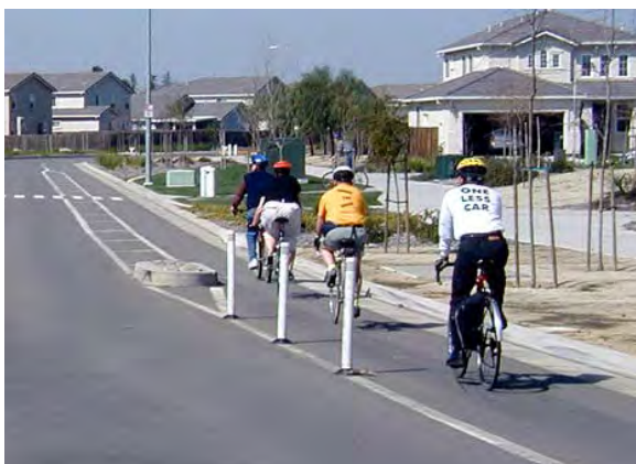
Buffered bike lane with vertical barriers
