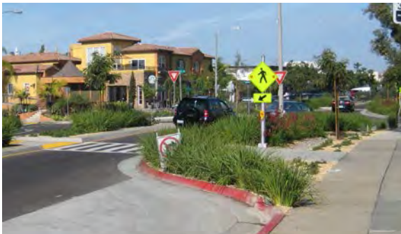
Curb bulbout at crosswalk with landscaping
