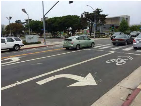
Shared bicycle/vehicle turn lane with sharrow markings
