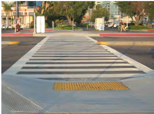
Crosswalk with ladder marking pattern
