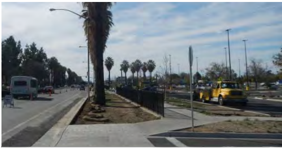
Pedestrian access from street into Walmart parking lot
