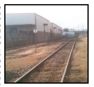
The rail steel track components include tie plates (which hold the rail to the wood cross ties), some anchors (which provide additional support for holding the rail to the ties), and spikes (holding the tie plate to the ties). The track is mostly single spiked plates with a few double spikes and even a third spike in some areas.
